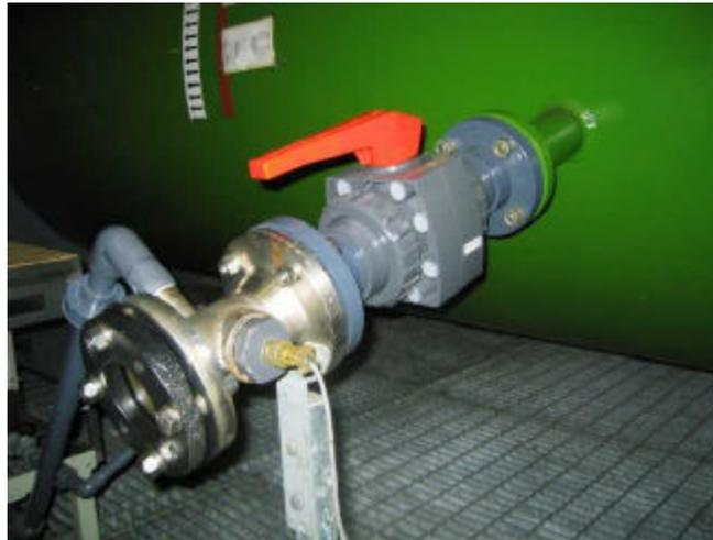
FIGURE 4 - Probe Tapping on Cooling Water Return Line
